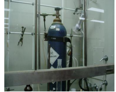
Poisonous gas being used within a fume hood, not an approved ventilated gas cabinet.
