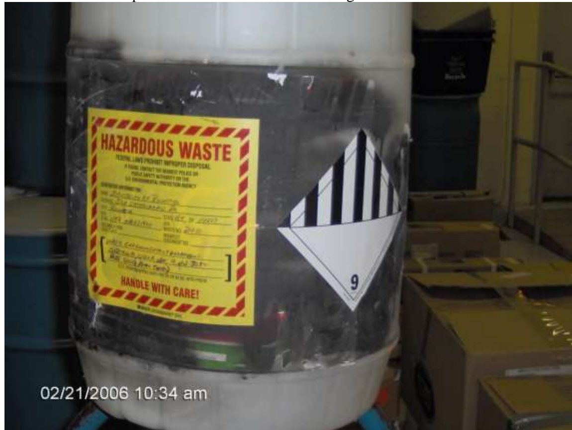
Figure 10 - Properly Labeled Plastic Container for the Collection and Transport of Used Photo Fixer
